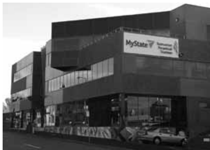
New green-star rated building at 137 Harrington Street, Hobart
